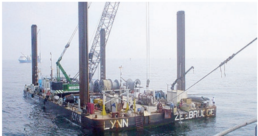
Cable laying within an offshore windfarm
