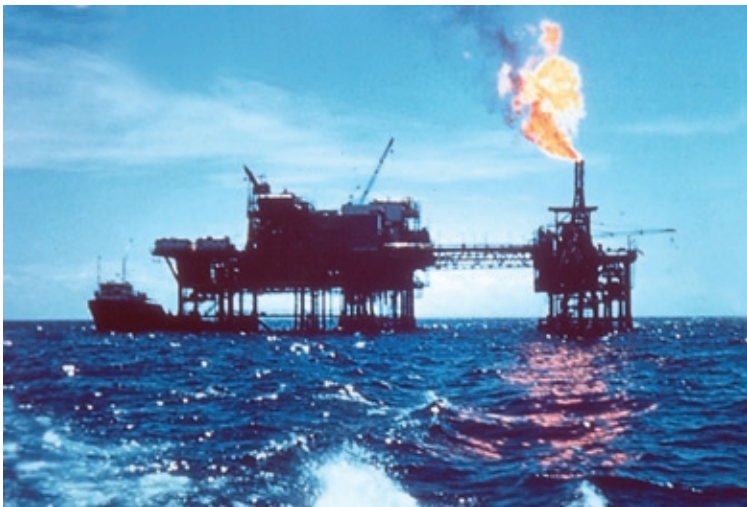
Offshore production platform in Indonesia, with power supply through a submarine cable
