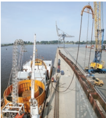
Transfer of a submarine cable into a laying vessel
