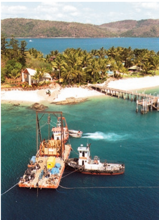
Landing a submarine cable at shore of an Australian Island
