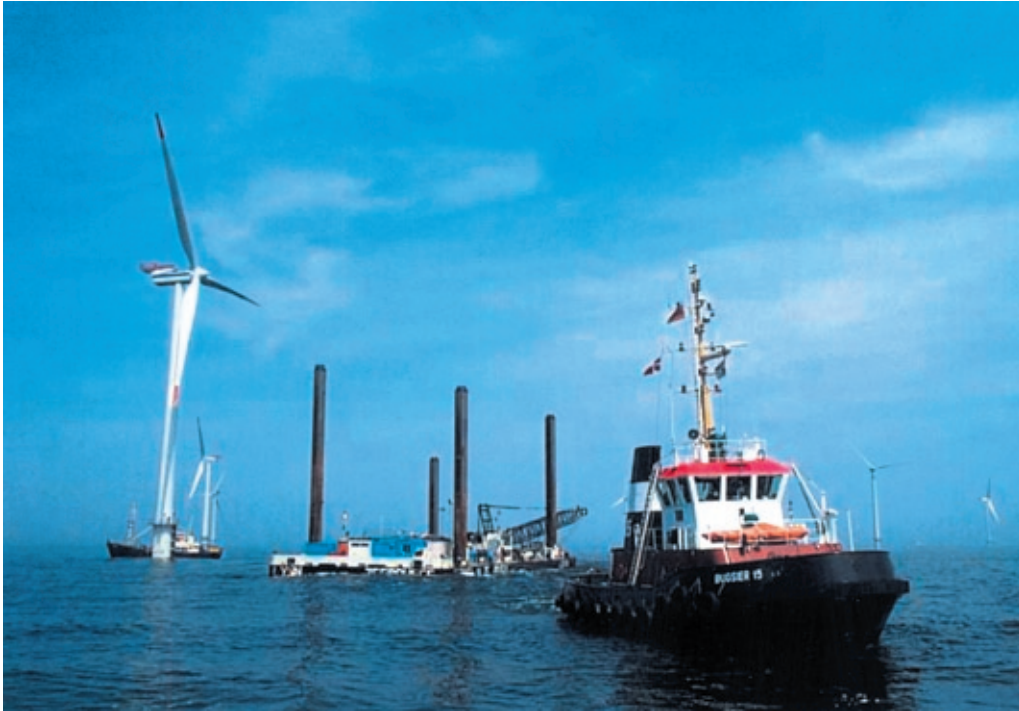
Laying of inter turbine cables for Horns Rev offshore windpark, Denmark
